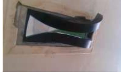
5. Lubricating the new gasket with Plumbers Grease, Vaseline, Silicone spray, WD-40 or dish washing liquid will help it slide into place easier. The lubricants also prolong the life of the gaskets and should be applied once or twice a year.
