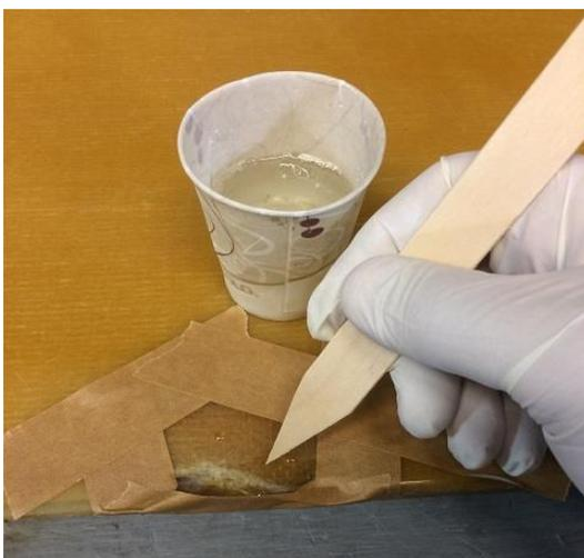
*Use a tongue depressor to drizzle the epoxy into the repair*
